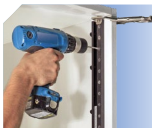
Drilling for placing shelves.
