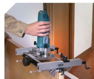
Making the first recess on the door.
