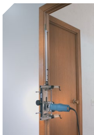
Making the second recess on the frame.
